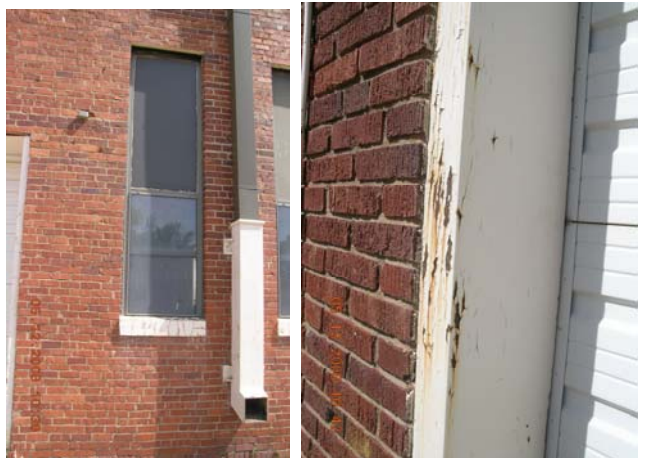
Photo: 10) Downspout/Oh Door Frame Pre Remediation
