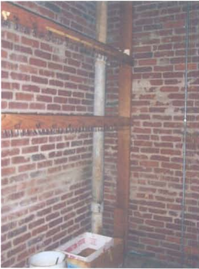
Hot Water Heater Transite Exhaust Pipe
