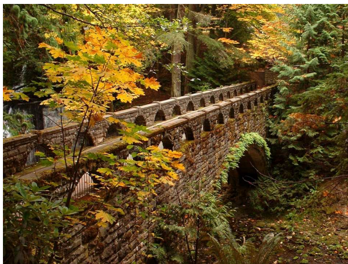
Whatcom Falls Bridge, Photo by GJ Beide
